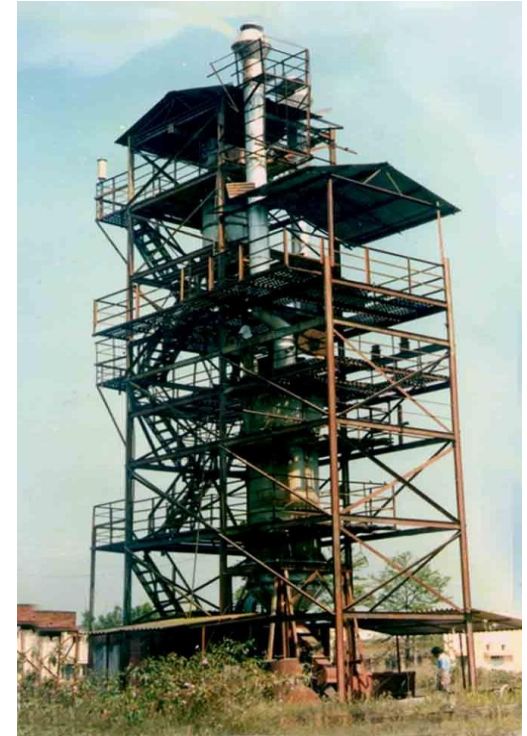
✓ VSK cement plant
